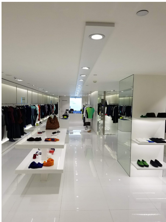
Application on a Retail Shop DOUBLE line series applied in ceiling and shelves SMD5050./ Serie DOUBLE LINE instalada en estanterias y techo.
