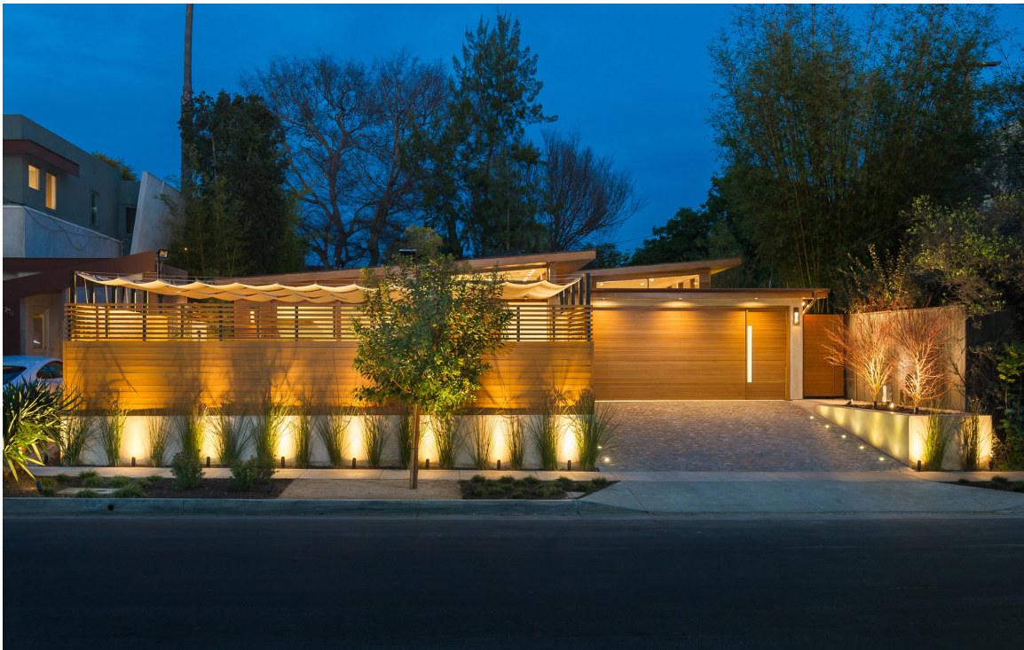
COMMERCIAL AND RESIDENTIAL OUTDOOR, Spike Spot Light series, reference SS4490 8W, a perfect spike spot light for outdoor illumination .
